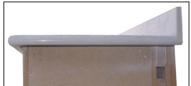
The result is a neat, uniform and evenly spaced trimmed bullnose bottom edge along the entire run.
