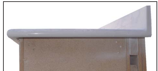
The result is a neat, uniform and evenly spaced trimmed bullnose bottom edge along the entire run.
